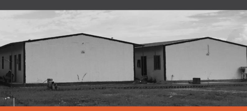
The term prefab is used to distinguish this process from the more conventional construction practice of transporting the basic materials to the construction site where all assembly is carried out.
